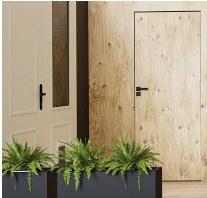
Door with a concealed door frame / Door with a flush wooden door frame (concealed hinges)
